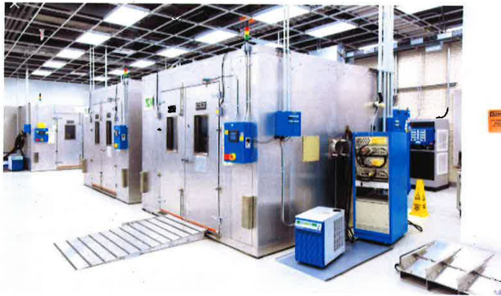
General Motors 100kW Test Lab – Commercial Off-The-Shelf Testing Chambers
