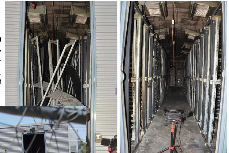
Surprise, AZ, USA, 2019 BESS in prefab building. Battery thermal runaway with explosion.
