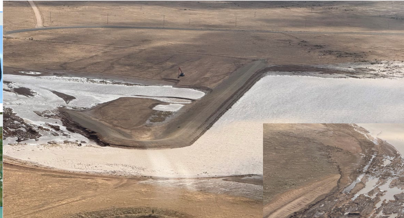
Zuber Hollow Site 1 (13 Mile Draw) Dam
