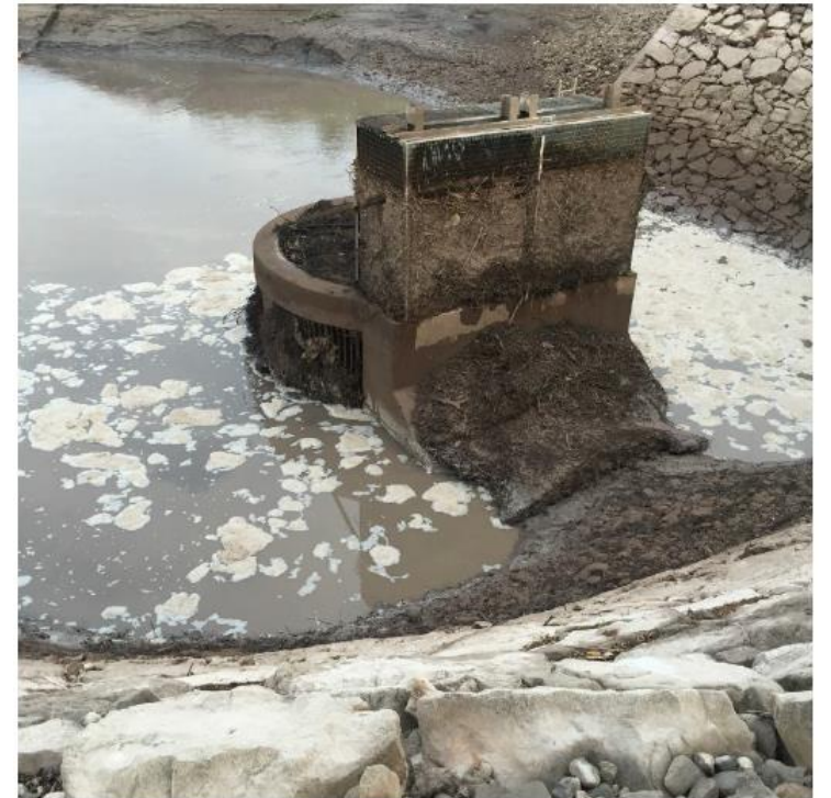
Caballo Reservoir intake structure, 2024
